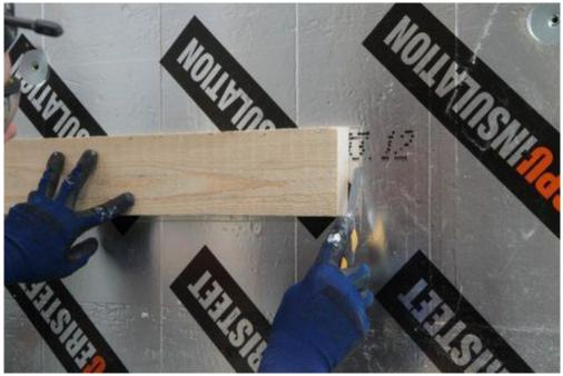
If the framework for the sauna benches is designed to be supported by the walls, cut a piece of insulation slightly larger than the bench support from the place at the support will be attached.
