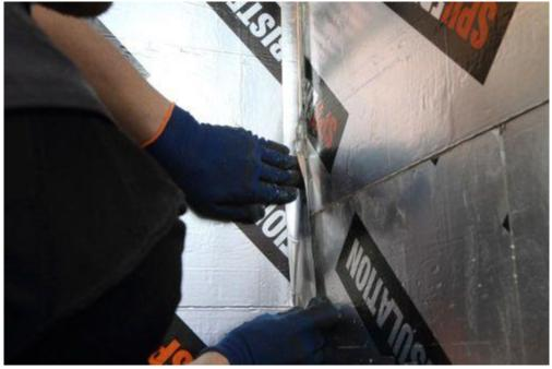
After you have removed any excess sealing foam, tape all seams with aluminium tape. You must also tape the seams of the lead-ins and benches as well as the heads of all fasteners.
