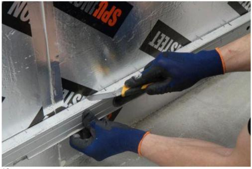
The tile skirting for under the sauna panels is installed directly on the surface of the insulation board. Before starting the work, measure the height of the upper edge of the tiling.
