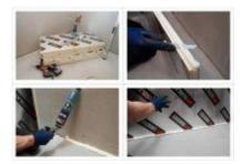
SPU Sauna is a 30-millimetre-thick insulation board with an aluminium laminate surface and tongue-and-groove edging on all sides. SPU Sauna is the most efficient insulation board for insulating sauna walls and ceilings. It is also an excellent material for insulating a suspended bathroom ceiling. SPU Sauna is suited to both stone and timber structures.
