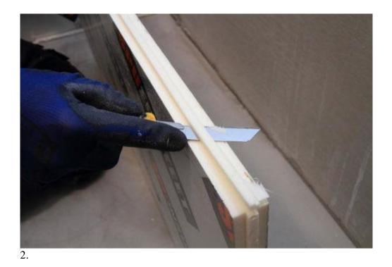
Before installation of the board, cut off the tongue edge with the Stanley knife.
