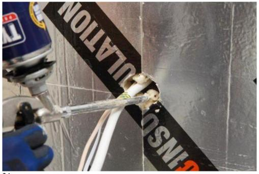
Once you have installed the ceiling boards, the openings for the ventilation ducts and tubes must be sealed with sealing foam.
