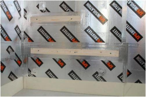
Apply sealing foam and tape the seams between the support and the insulation layer. Also ventilation ducts on wall can be installed in SPU Sauna insulation layer. The sealing is made in the same way: foam and tape. The duct can also be installed on either side of SPU Sauna in case there is enough room for it.
