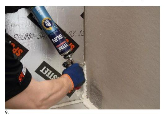
Apply sealing foam into the corners as well.
