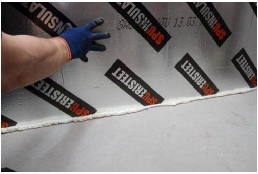
Install the first board horizontally with the female edge facing down and the code text on the board facing the sauna space. The date/code text of the insulation board should face the sauna space during installation.
