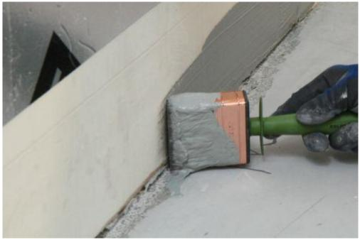
Install the moisture barrier against the SPU Sauna. Tile the plinth normally to the surface of the insulation board.
