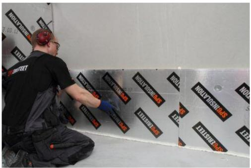
When sealing foam has been applied to the tongue-and-groove, install the next board. The tongue-and-groove makes the seams between boards tight.
