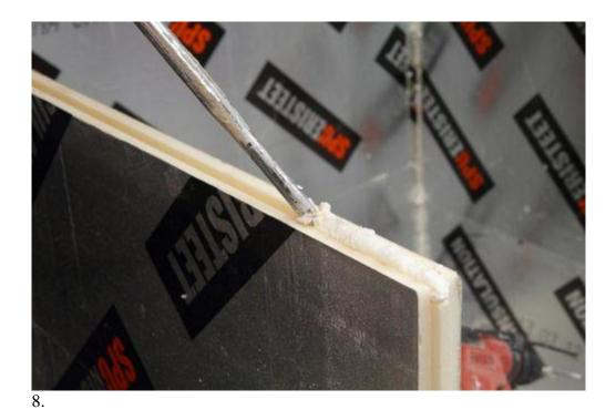
Apply sealing foam into the tongue-and-groove of the board before installing the next board. An amount of sealing foam that fills the insulation board's groove edge is sufficient.
