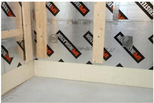
The aluminium paper is easiest to remove from the side of the board on which the code text is printed.
